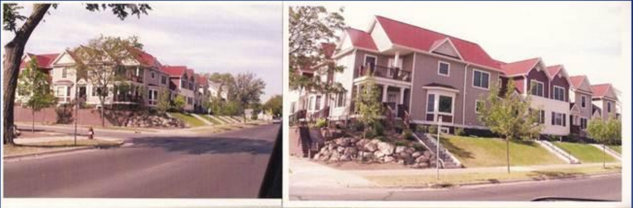
Franklin Station Town Homes After
